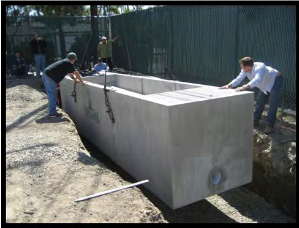
The Modular Wetland Is Lowered Into Place
