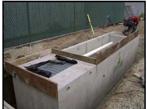
The Curb and Gutter Form is Built in the Appropriate Configuration Along The Outer Perimeter of the Modular Wetland
