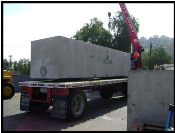
Pre Assembled Modular Wetland System Loaded At Manufacturing Plant
