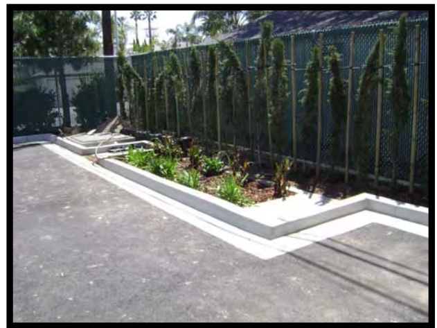
Pavement is Pored And Vegetation Is Planted. Once The Site Is Stabilized And Cleaned The System Is Ready to Activate.
