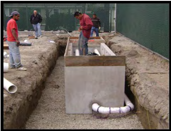
Appropriate Size Outlet Pipe Is Connected Into The Modular Wetland Systems Discharge Chamber And Appropriately Routed
