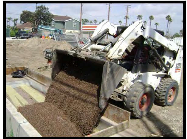
The Modular Wetland Should Be Filled To The Top And Covered With Plastic Until Activation After The Site Is Stabilized
