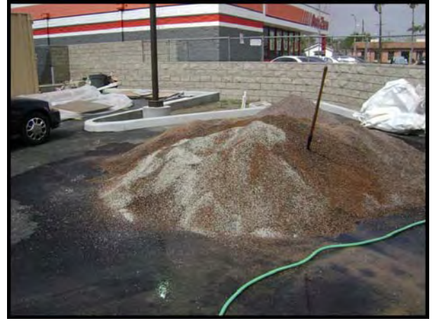
The Filter Media Is Mixed Per Manufactures Recommendations And Is Now Ready For Installation
