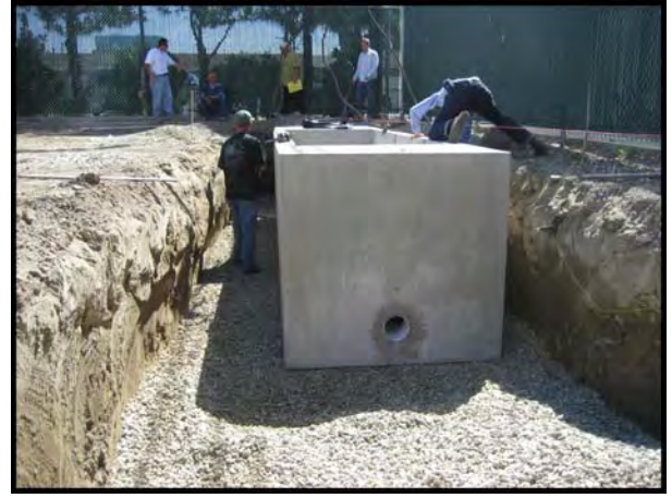
The Modular Wetland Is Set Into Place and the Lifting Knuckles Are Detached. Elevation Should Be Confirmed
