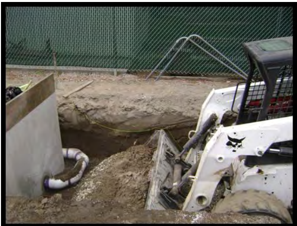
The Area Around The Modular Wetland Is Carefully Backfilled
