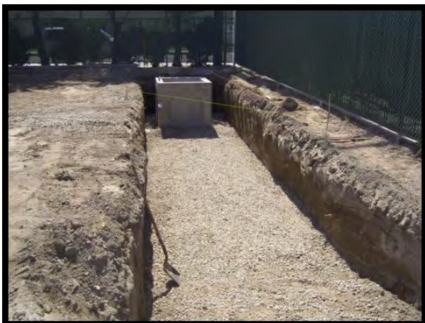
The Hole Should Be Excavated Prior To Delivery And To The Appropriate Elevation. The System Is To Be Installed On 6" Of Level Rock Backfill
