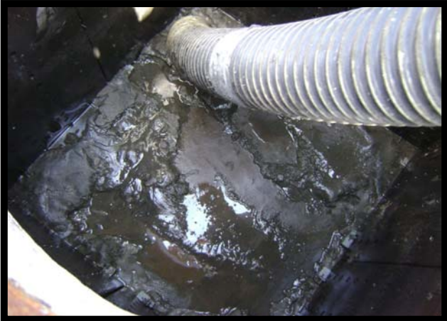
Sediment Chamber Is Vacuumed Clean Of All Accumulated Sediment And Associated Pollutants.
