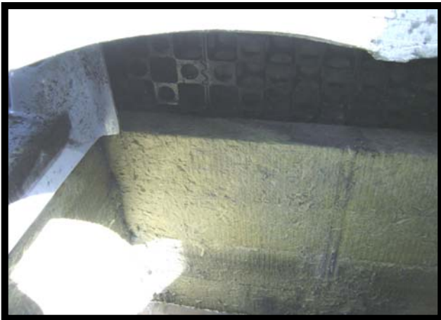
Washed Or New Media Is Now Ready For Use. If Media Was Replaced, Old Media Will Need To Be Properly Disposed Of Properly.
