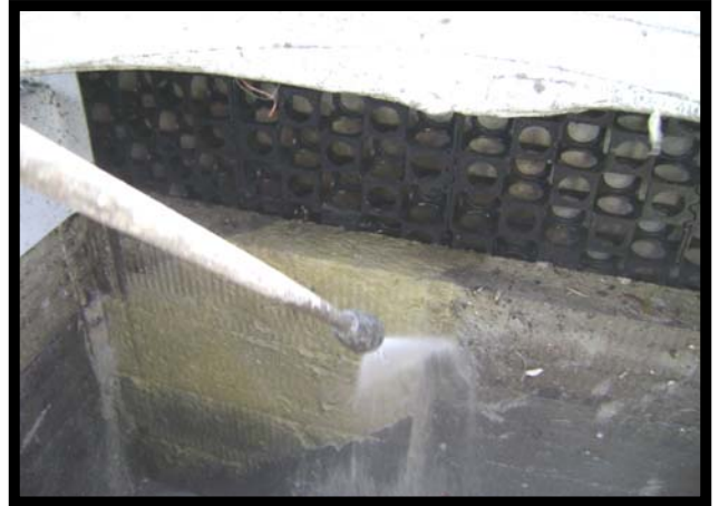
Media To Be Power Washed To Reveal Extent Of Clogging. If Only Surface Is Clogged, Media Can Be Re-Used Once. If Clogged Replace With New Media Blocks. Remove and Replace.
