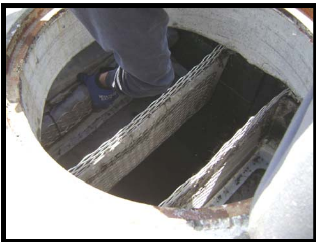
Replace Catch Basin Filters.
